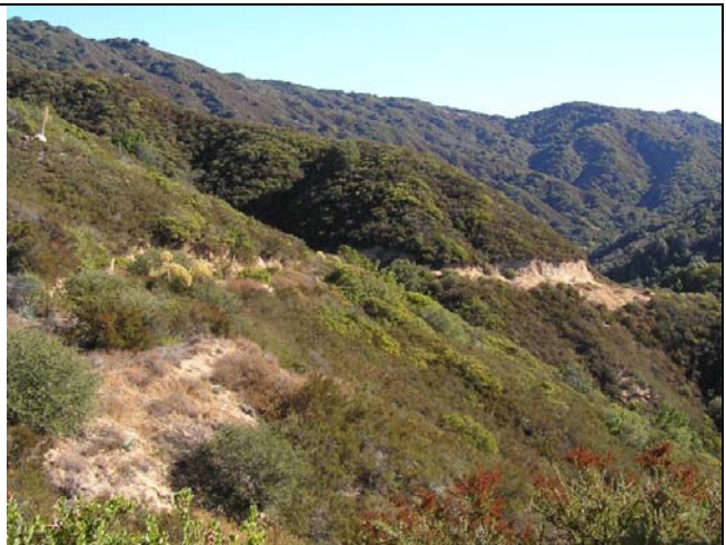
View of decommissioned spur road immediately to the right of junction with Garrapata/Wildcat Ridge. Note tall road cut and evidence of landslide below the head wall of the decommissioned road.
