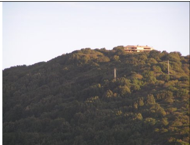
Power lines that span Garrapata Canyon are below the new home west of Twin Peaks. This structure has been built since the August 2004 photo on page 14.
