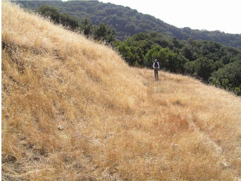
Decommissioned roadbed in Grassland area along the Lopez-Perez Loop southwest of the hunt camp. This stretch of road does not appear to have had noticeable "treatment" related to road decommissioning, however the simple act of ripping the compacted roadbed could have led to invasion of weedy annuals, as is depicted in this photograph.
