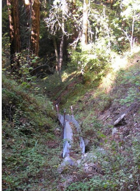
Open culvert constructed of corrugated tin along old roadway down into bottom of Wildcat Canyon. Metal T-posts supporting downstream end of culvert have not rusted, indicating their relative youth compared to other cultural features in the bottom of the canyon.
