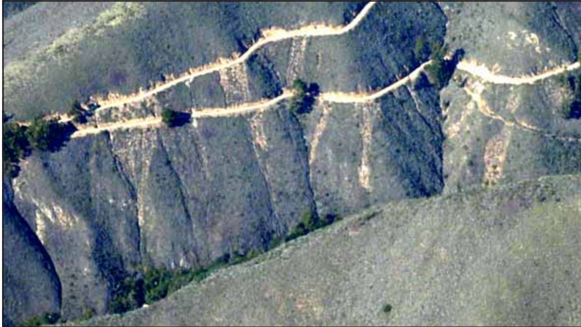
Figure 18: Sediment aprons shed from side-casted road cut material in Joshua Creek Watershed. Photo: D. Smith October 31, 2004.
