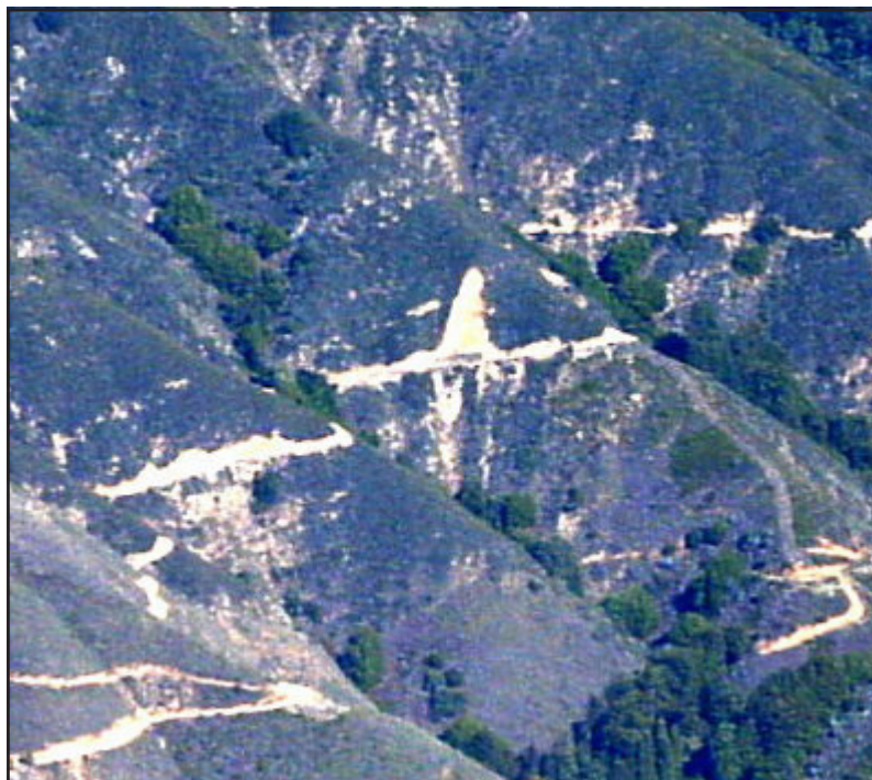
Figure 19: Shallow soil slip and sediment aprons along the roads in Joshua Creek Watershed. Photo: D. Smith October 31, 2004.
