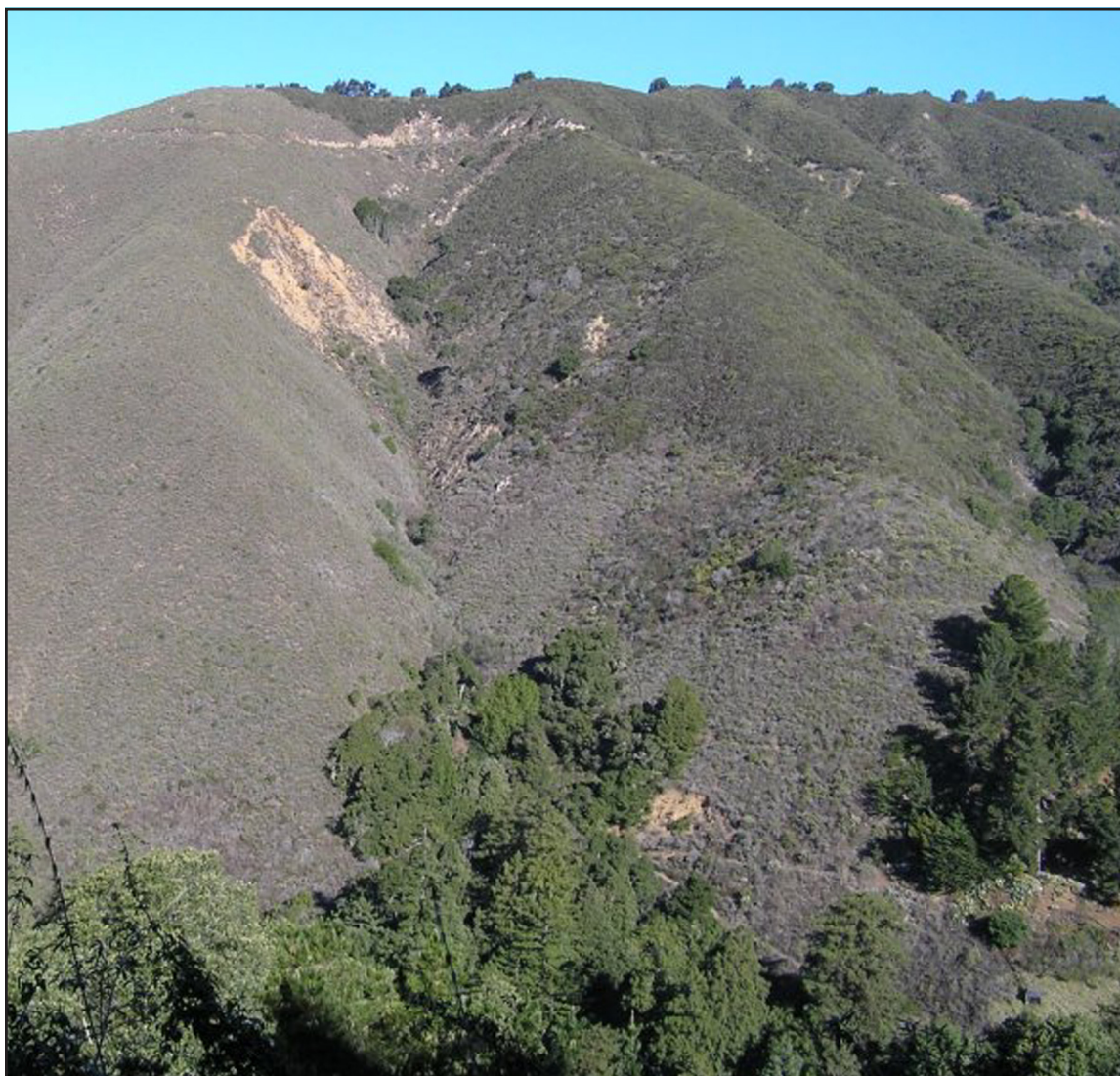
Figure 21: Portion of Little Horse Ranch road decommissioned in 1991 is seen near top of ridge. Photo: N. Nedeff, 2006
