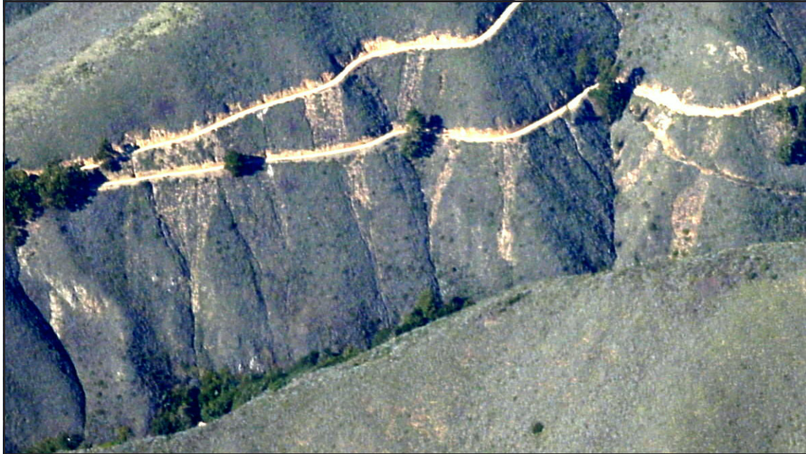
Figure 18: Sediment aprons shed from side-casted road cut material in Joshua Creek Watershed. Photo: D. Smith October 31, 2004.
