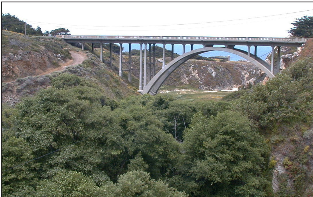
Figure 6: Same view as Figure 5. Photo: N. Nedeff July 2004.
