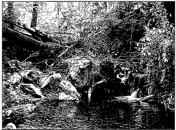
Post Creek near park boundary. Numerous logjams and passage barriers exist between PCRM 0.15 and a large landslide toe at PCRM 0.38..
