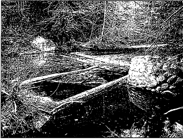
Old diversion dam site. (PBSRM 0.13) This existing structural grade control feature is one of 8 old instream grade controls that affect channel width/depth dimensions in PBS.
