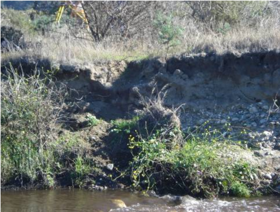
Figure 32: Detail of weak floodplain deposits underlying eroding terrace (November 2008).
